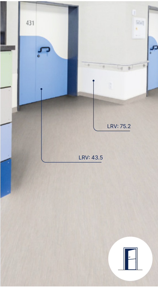
LRV differential of Wall/Door >30 Points = Public Door
