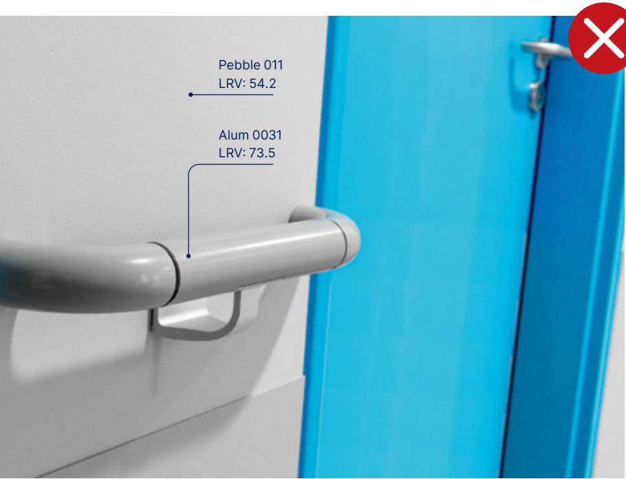
LRV differential of Wall/Handrail <30 Points
