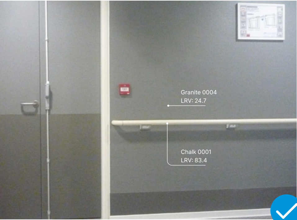
LRV differential of Wall/Handrail >30 Points
